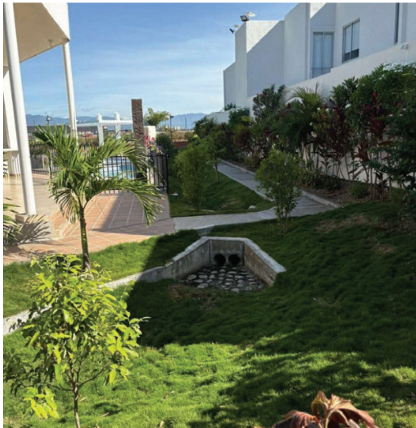
The Arezzo Condominium and surrounding sustainable drainage systems. Image: Condominio Arezzo
