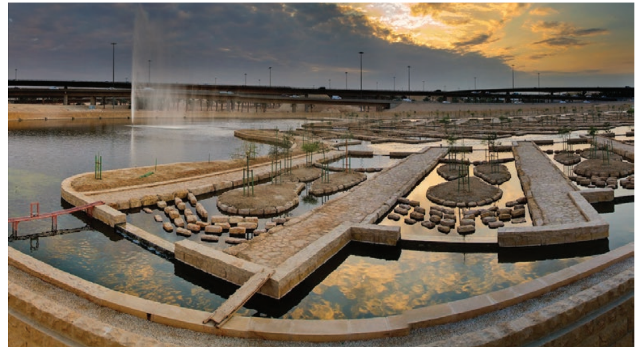
The bioremediation facility relies on a food-chain-based approach in which primary producers (algae and higher-order plants) and consumer organisms (fish, birds, and insects) break down urban wastewater components. Image: Riyadh Bioremediation Facility
