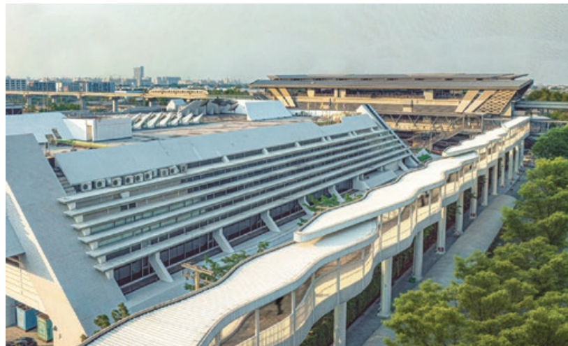
Covered walkways with rain chains and comprehensive drainage systems channel rainwater to rain tanks and a retention pond, achieving zero-runoff discharge. Image: Landprocess
